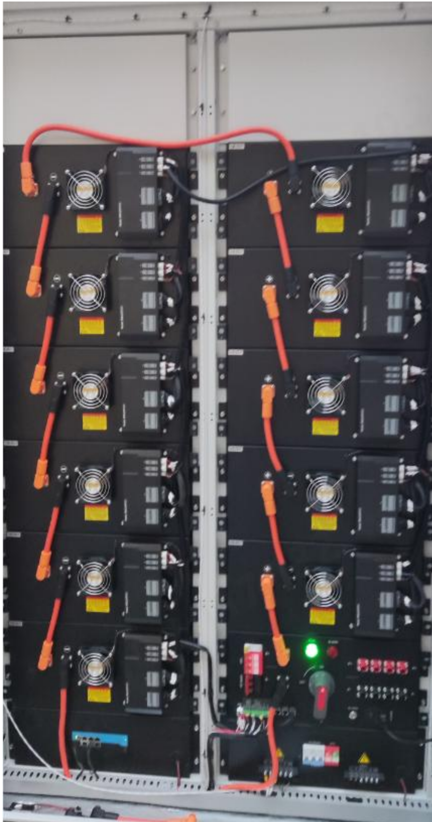
Fig. 3-7 Power Wiring Diagram
